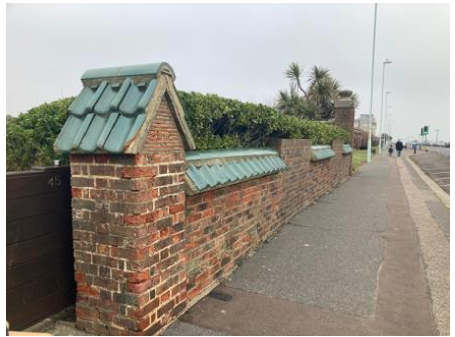
Figure 16: Brick boundary walls with green pantile capping
