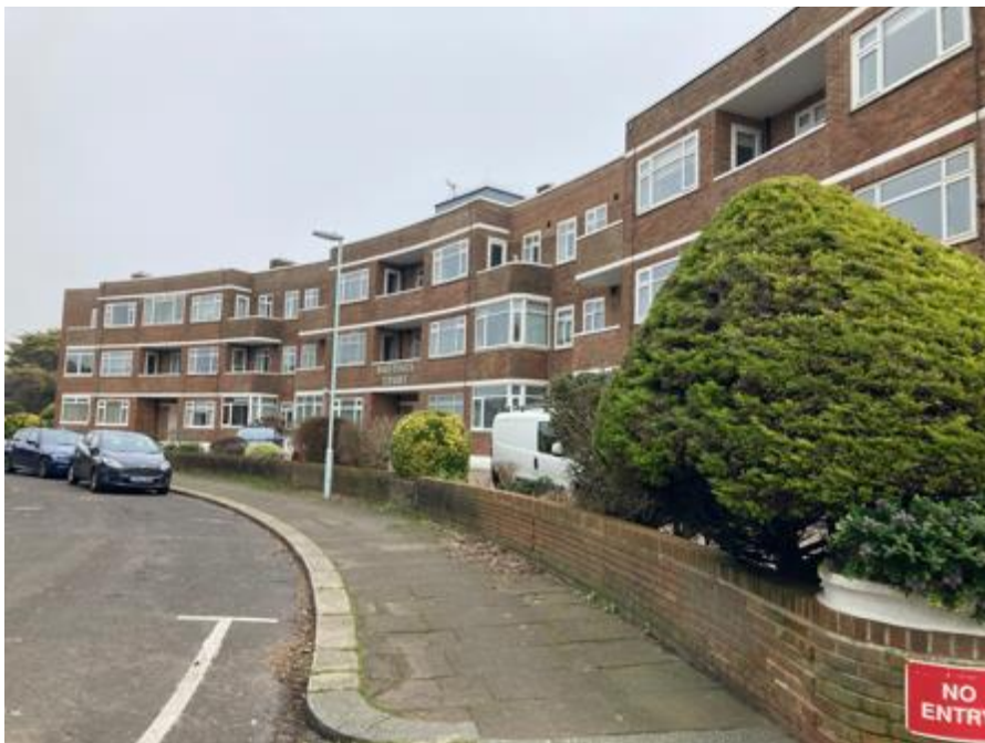
Figure 26: Hastings Court front elevation
