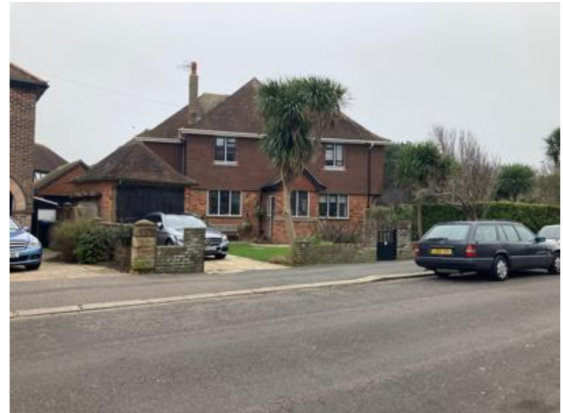
Figure 29: No.2 Dover Road
